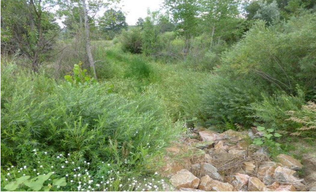
Players Crossing: PICTURE NO. 13: The Town of Castle Rock recently repaired and improved their portion of the retention pond where the Association's drainage channel enters the retention pond.
